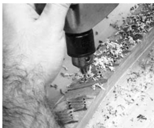
**Figure 444** Drilling epoxy out of bridge pin holes.
