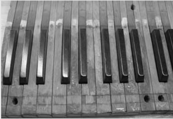
Figure 525 The person who removed ivories from these keys inadvertently pulled off wood strips from the front mortises. If the strips are not restored, the tops will click in those spots.
